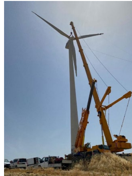
Tower under construction
