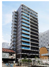
S-RESIDENCE Nihonbashi Qualier
