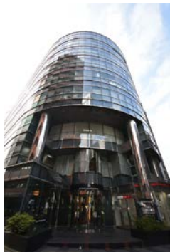
Hatsudai Center Building
