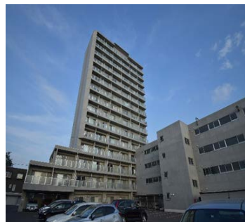
SAMTY Tower N26, ELM Kita26jo
